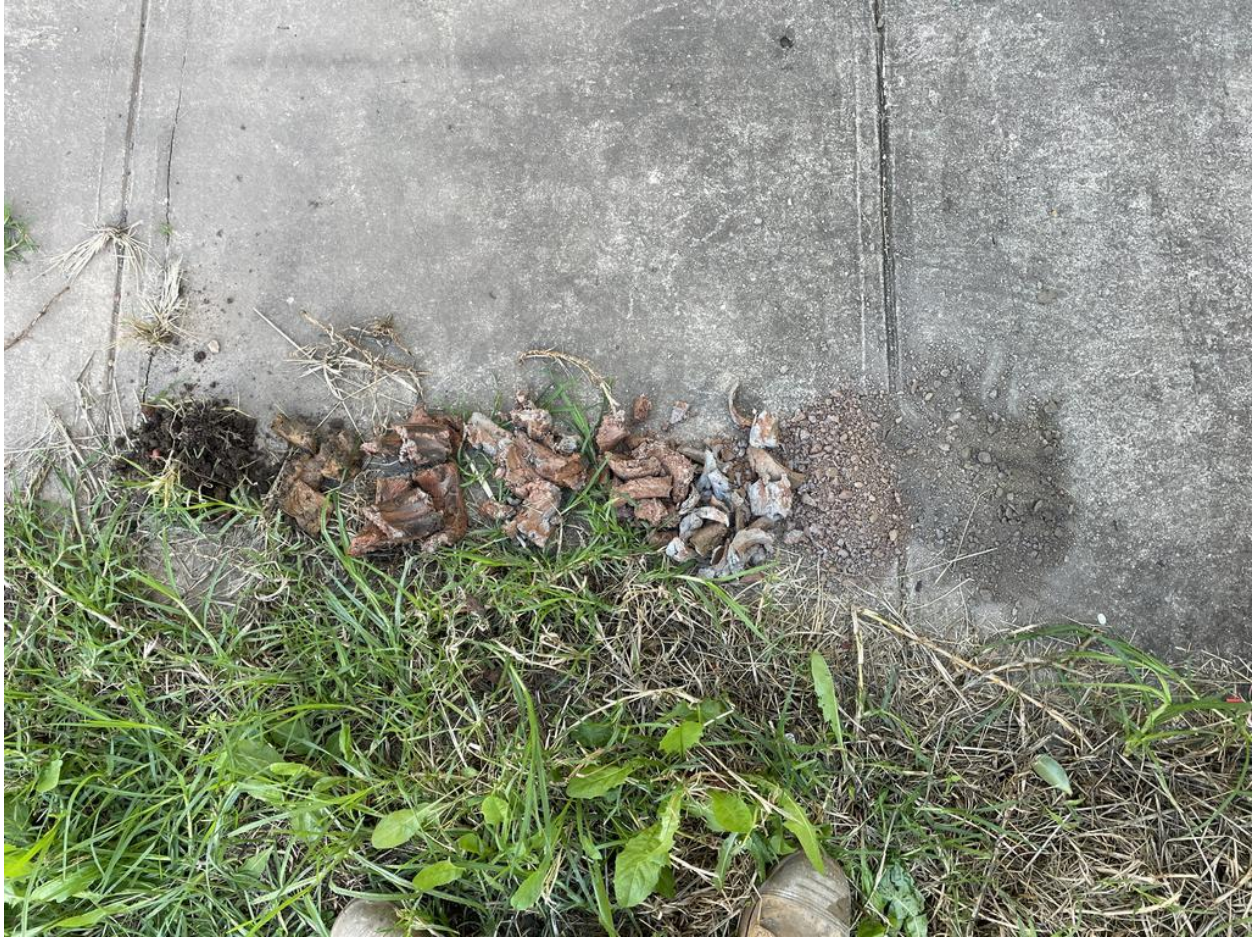
Subsurface Material - BH1
